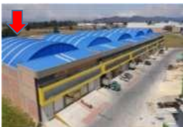
Bodega DELOGIC Bodega interna DELOGIC trasera
